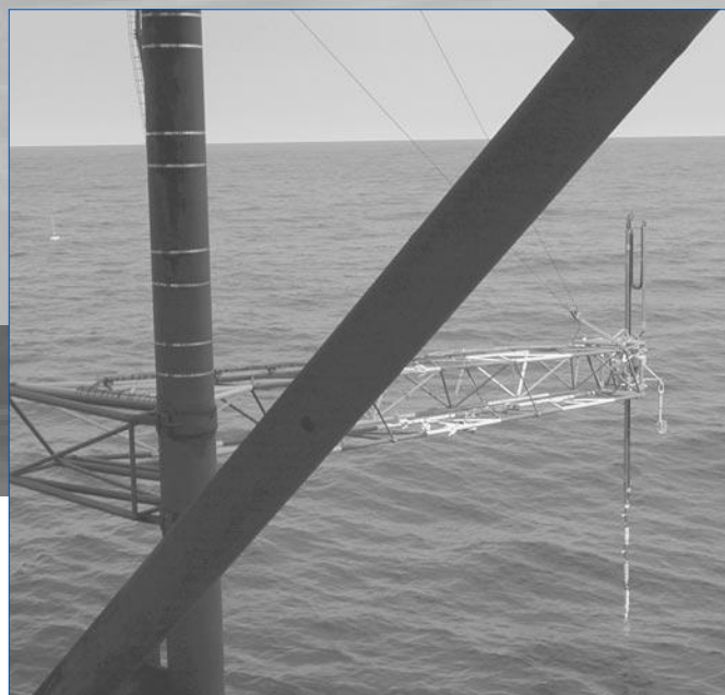
Figure 2. Photograph of the wave follower in action. The photograph was taken below the main body of Meetpost Noordwijk. The black structures in the foreground are part of the jacket construction that supports Meetpost Noordwijk, and to which the wave follower boom is attached.
